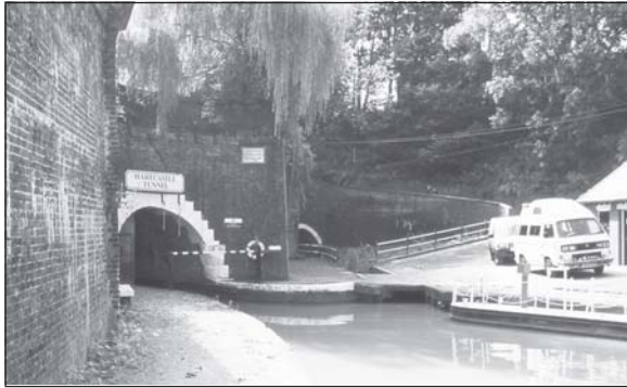
Harecastle tunnels today. In the foreground is Telford's new tunnel whilst the earlier one by Brindley, now abandoned, can be seen in the background. (Author)
