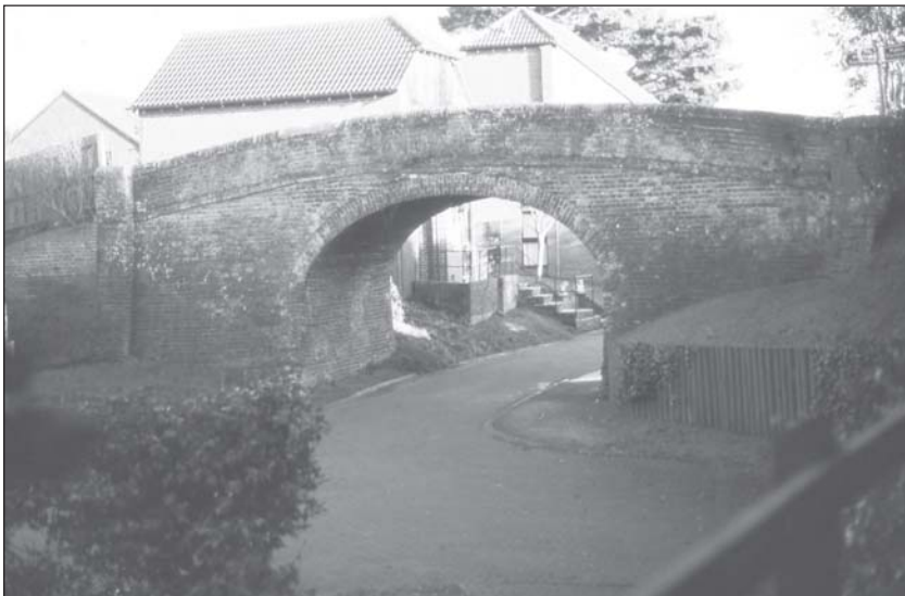
Tack Lee Bridge over the line of the former Portsmouth and Arundel Navigation, Yapton
