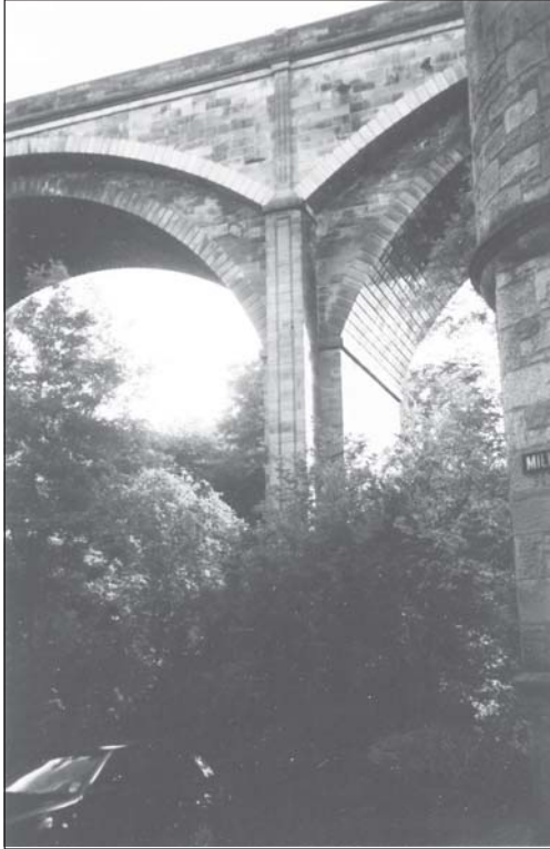
A detail of Dean Bridge in Edinburgh. The shallower arches carrying the footways are part of Telford's original design and not a later modification as might be thought. (Author)
