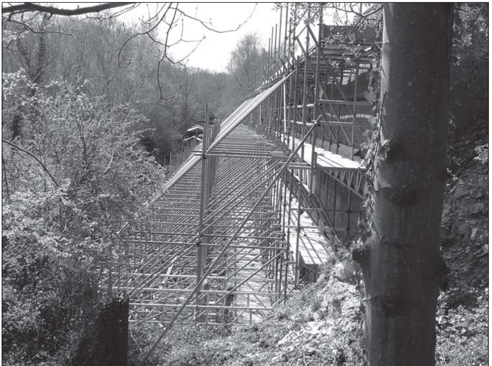
The scaffolding to the east of the De Witt Kiln
