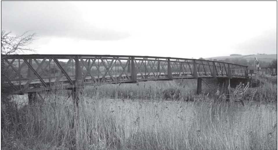
Fig 1 A long view of Offham Bridge looking east (Chris Bryan)
